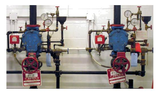
Shutoff valves for individual floors are located in every stairwell on each floor and at various locations in the parking levels.
