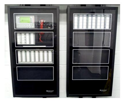
There are two remote annunciators located on the east wall of the 1st Floor fire control room (interior) and built into the east wall of the Pennsylvania Avenue entrance to the building that indicate in which zone the alarm was actuated.
