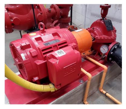
The fire pump supplies extra pressure to the standpipes and automatic sprinklers. The fire pump is activated automatically upon registering a water pressure drop in the system.
