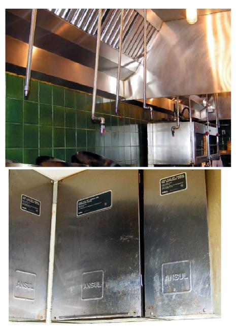
These systems are activated automatically when a fire occurs in a cooking appliance and a high-temperature fusible link melts or a heat detector is activated.
