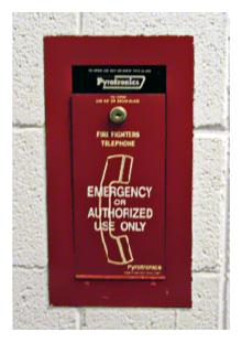
A tone at the fire alarm panel signals the evacuation control personnel that a person is on another phone within the office building. The phone has the characteristics of a party line, in that communication is not limited to just two persons.
